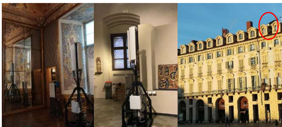
Figure 7-2: Installation for 5G indoor coverage in Sala Quattro Stagioni and Sala Acaja and rooftop antenna for the 5G outdoor coverage
